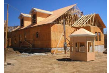
New town hall under construction
