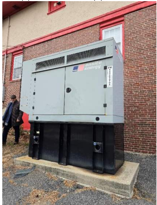
Photo 43: Diesel generator.
