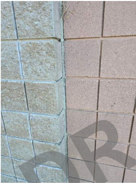
Photo 30: Failing masonry soft joint.
