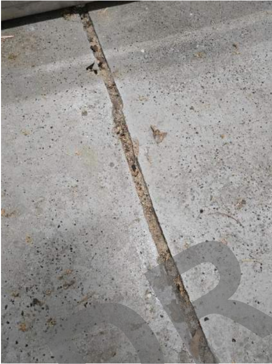
Photo 16: Concrete slab control joint.
