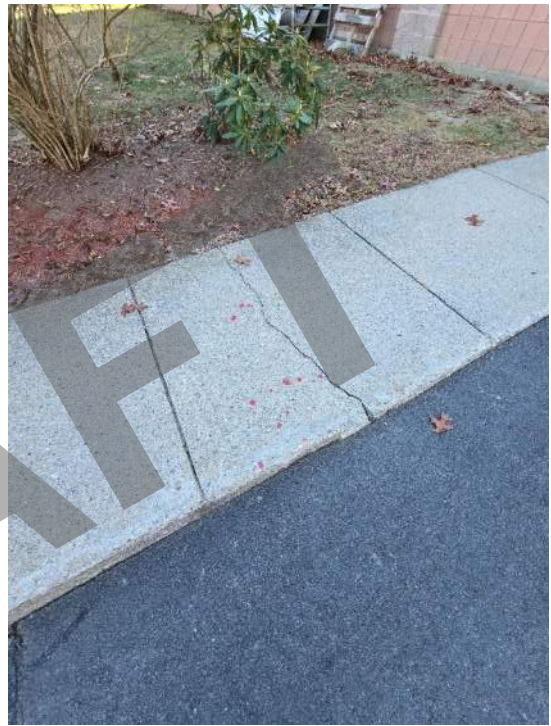
Photo 31: Cracking sidewalk.
