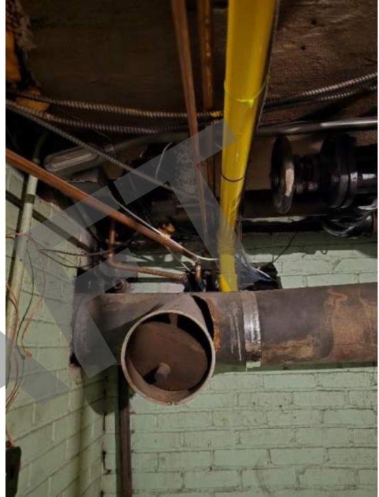
Photo 41: Abandoned ductwork/ Unsupported masonry penetrations.
