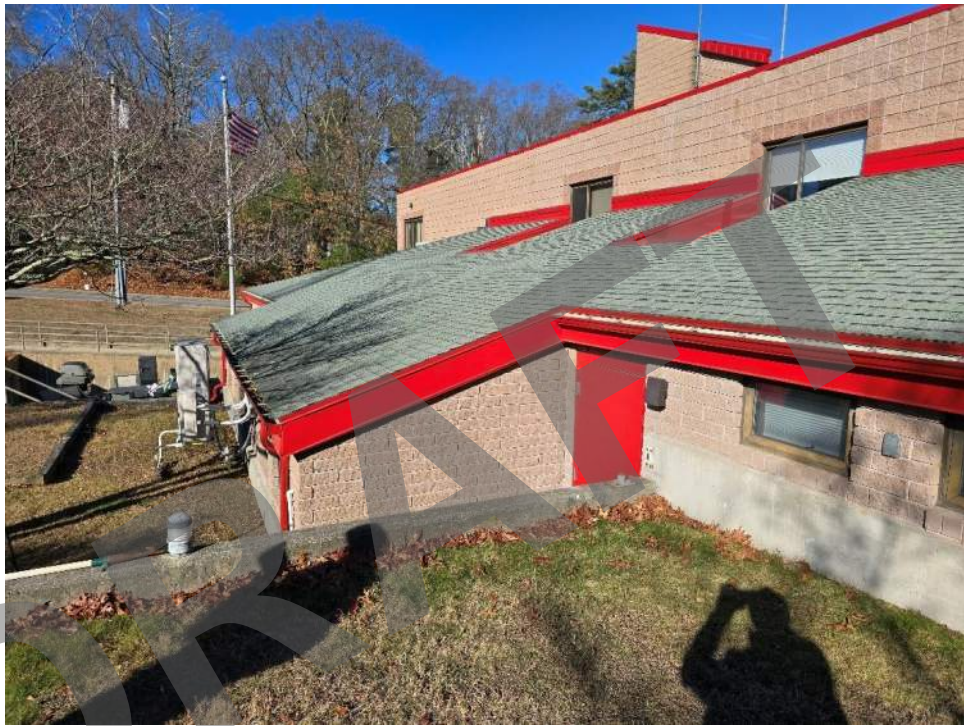
Photo 12: Asphalt Shingle Roof
