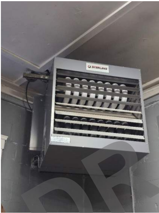
Photo 20: Unit Heater (gas fired).
