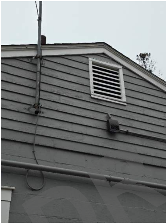
Photo 5: Wood siding and gable vent.
