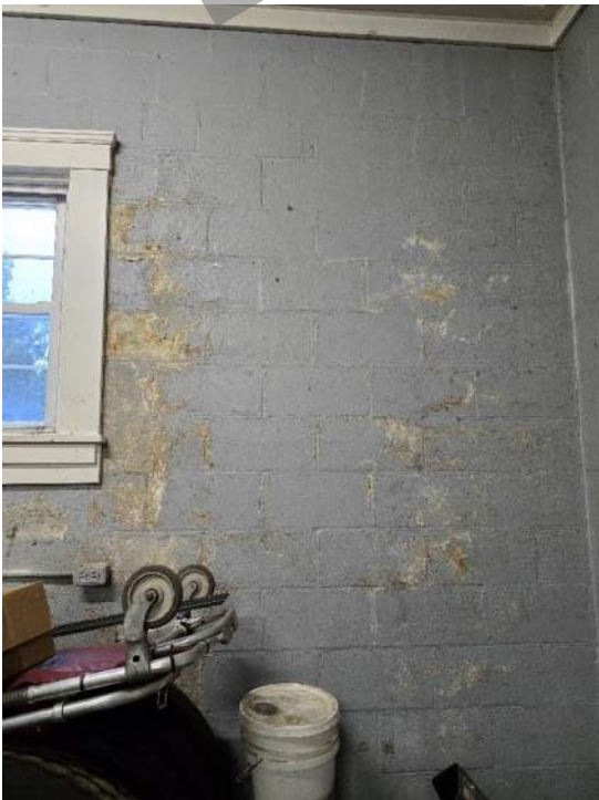
Photo 14: Exterior masonry wall staining.
