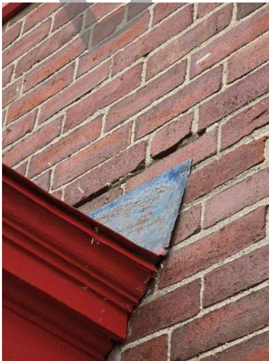
Photo 10: Side canopy – missing counterflashing.
