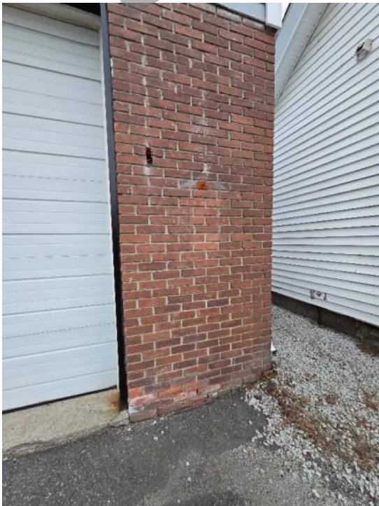
Photo 7: Masonry cracking.
