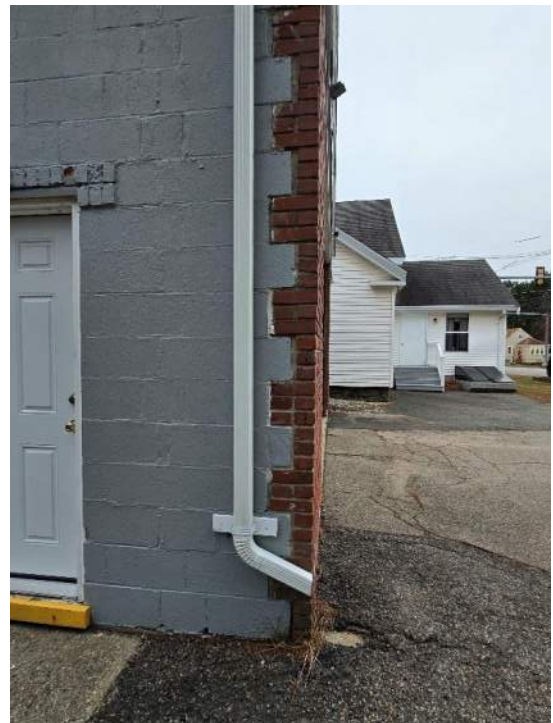
Photo 11: Building joint and downspout.
