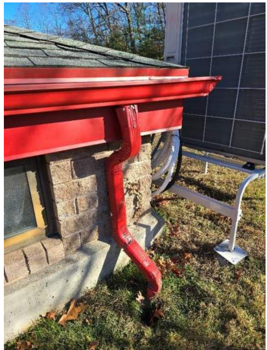
Photo 25: Low roof gutter and rainwater leader.
