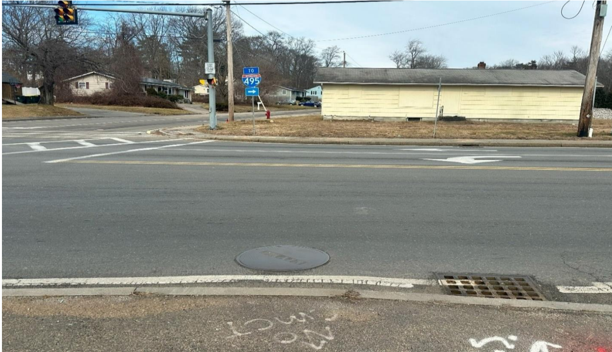
Sta. 13+00. Stormwater system 2. Hartford Avenue (Route 126). Two stormwater drainage catch basins are located along both sides of the curbline on Hartford Avenue (Route 126). Stormwater runoff is carried along the existing curb to existing catch basins. System 2 flows south along North Main Street (Route 126).
