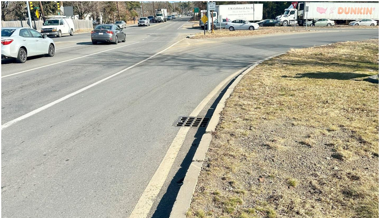
Sta. 22+50. Stormwater system 3. One drainage catch basin located at the curb line on Hartford Avenue (Route 126) entering on ramp of Interstate 495. Stormwater runoff flows east along Hartford Avenue (Route 126).
