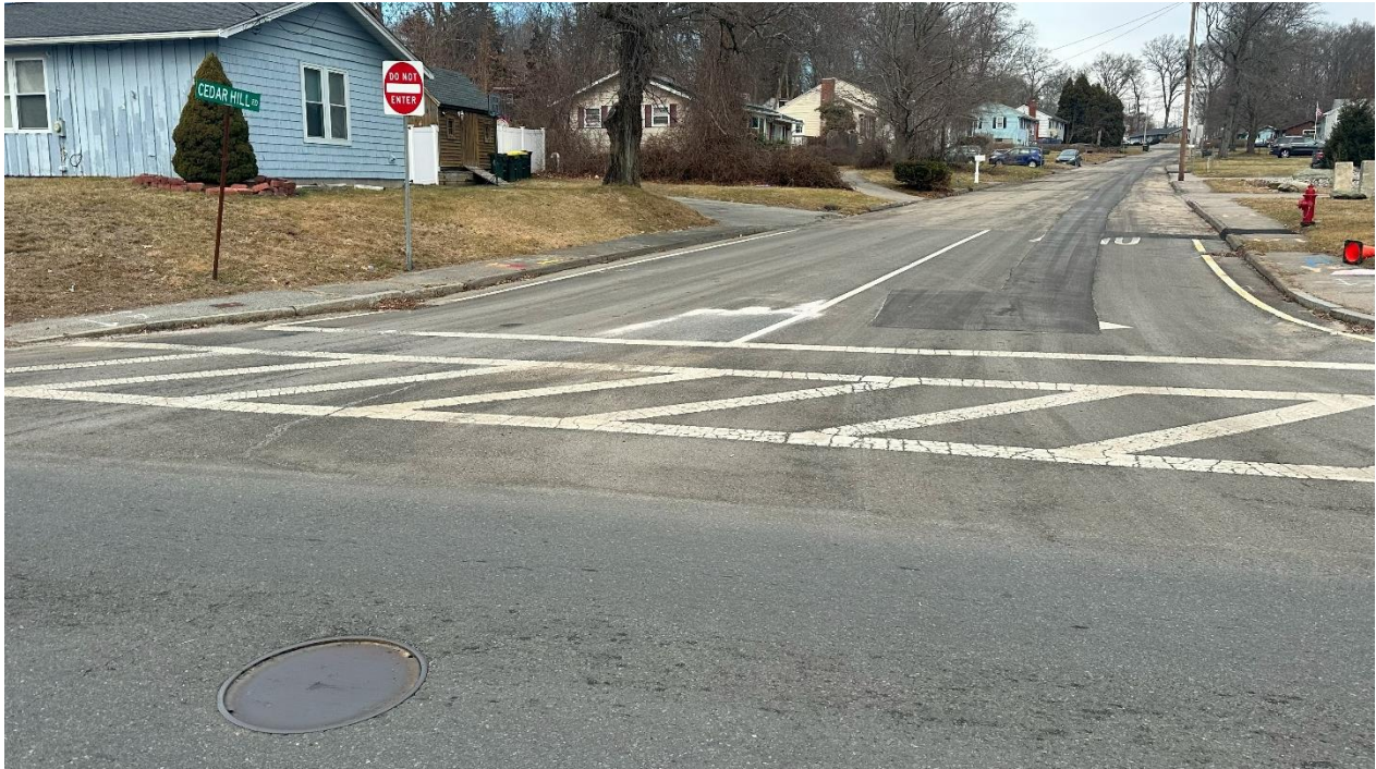
Sta. 12+00. Beginning stormwater system 2. View looking north along Cedar Hill Road. Two drainage catch basins located curbside capture stormwater flows along Cedar Hill Road. System 2 flows south along North Main Street (Route 126).
