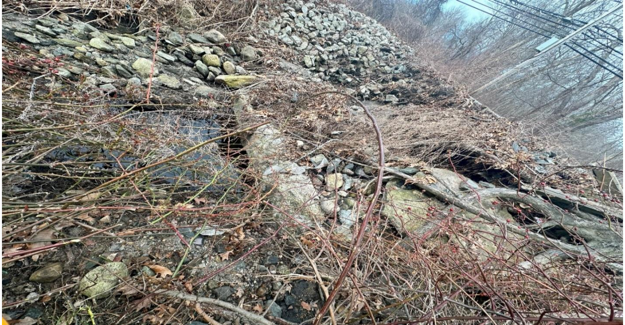
Sta. 5+30. Outfall end of Stormwater system 1. 18" RCP masonry headwall located at the bottom slope at the south side on Hartford Avenue (Route 126). Stormwater flows downstream. Note: Poor condition of masonry headwall and extensive bank erosion because of stormwater flows at roadside country drainage.
