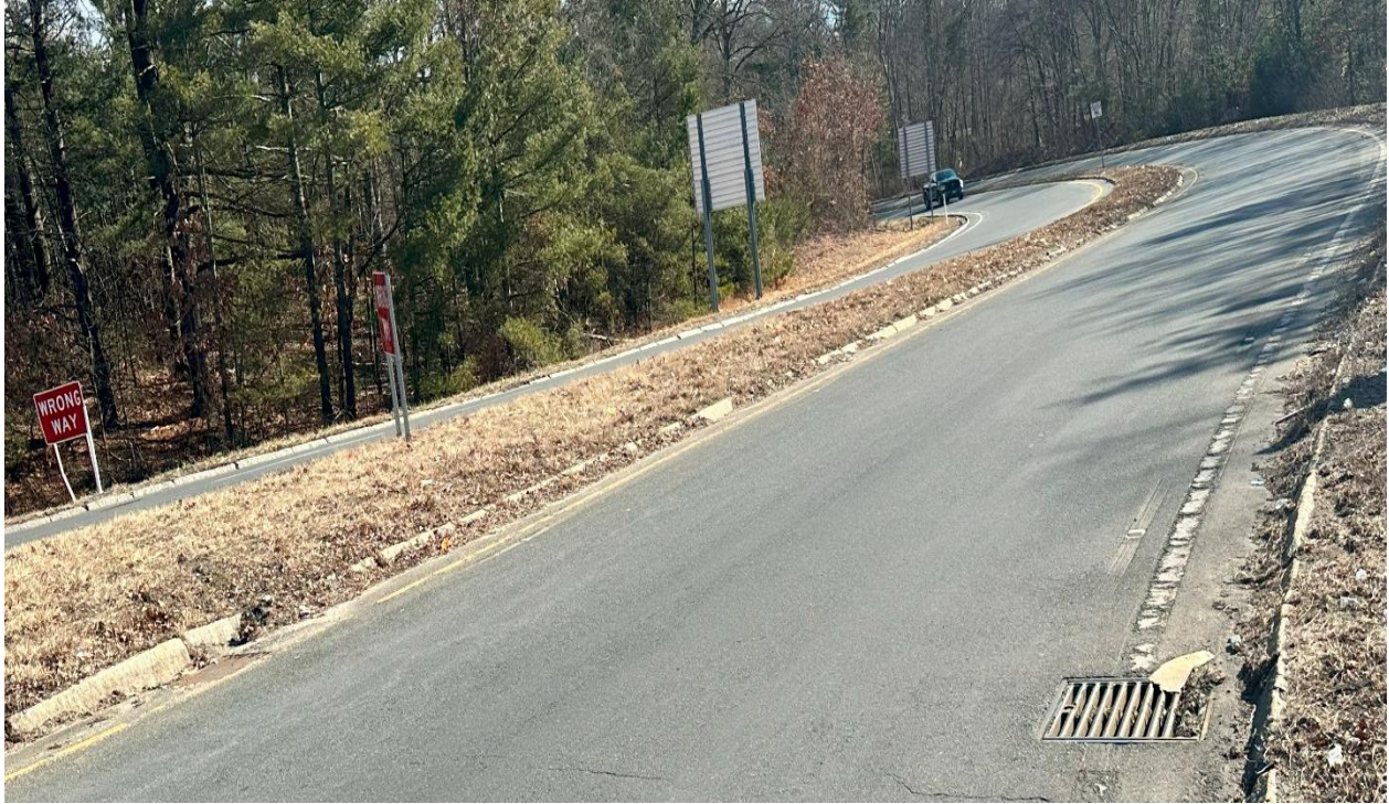
Sta. 12+00. Beginning of Stormwater system 4. View looking south along Interstate 495 southbound on-ramp. Two catch basins located along curblines capture stormwater runoff. System 4 flows south along the ramp.
