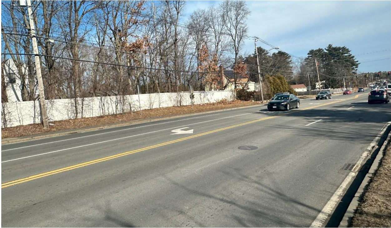
Sta. 20+00. Stormwater system 3. Hartford Avenue (126) looking east. Stormwater drainage structures are located at both curblines. Stormwater flows east along Hartford Avenue (Route 126).
