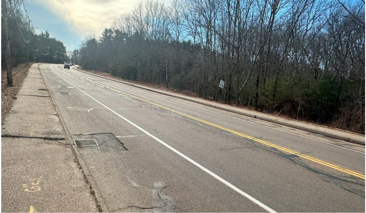
Sta. 93+00. Stormwater system 2. View looking south along North Main Street (Route 126). Three catch basins located along both curblines capture stormwater runoff.
