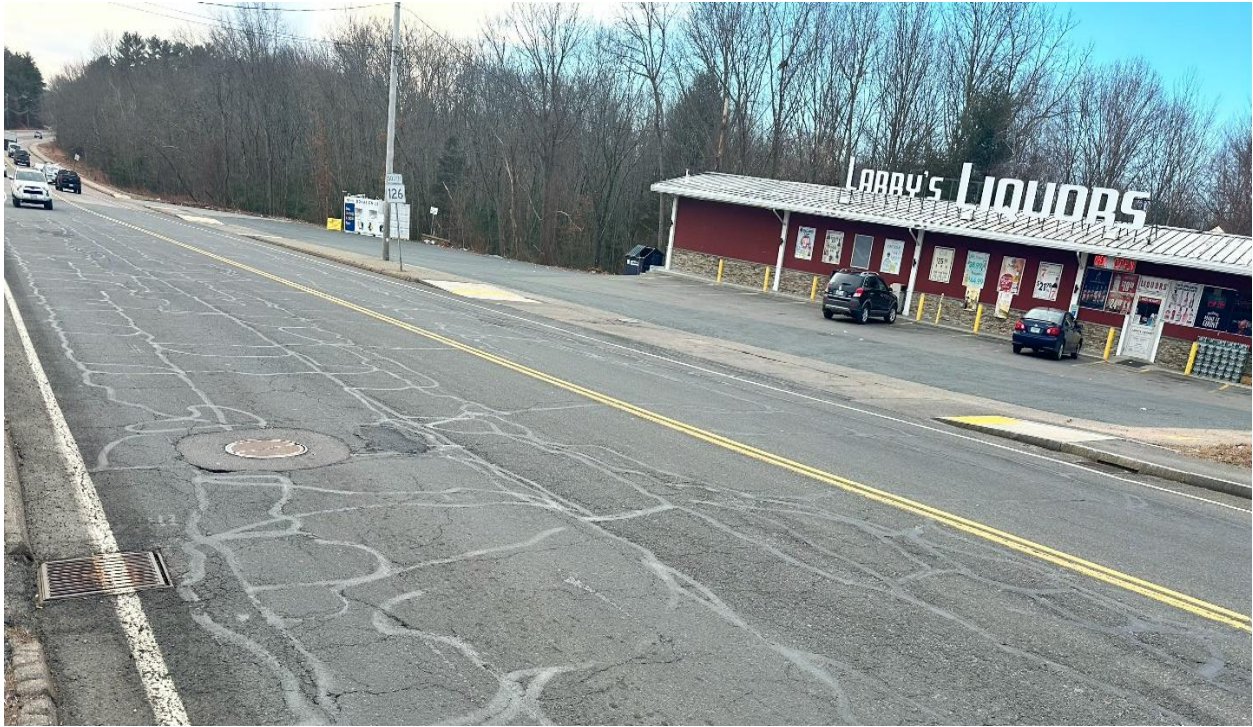
Sta. 98+20. View looking south along North Main Street (Route 126). Stormwater system 2. Two drainage catch basins capture stormwater flowing south downhill along curbside on North Main Street (Route 126).
