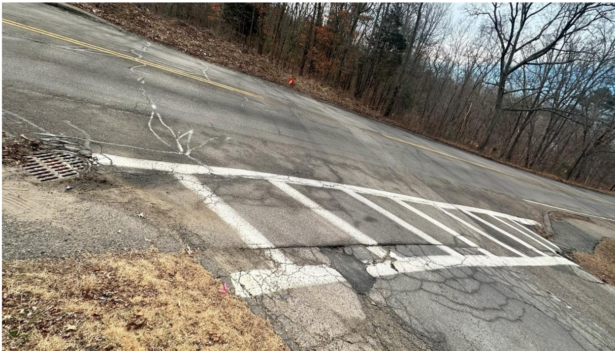
Sta. 9+19. Stormwater system 1. Two catch basins located curb side at intersection of Hartford Avenue (Route 126) and Arrowhead Road. System 1 flows west along Hartford Avenue to Farm Road.
