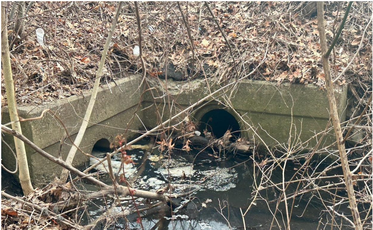
Sta. 5+50. Outfall of stormwater system 1 12" RCP. Inlet 18" RCP cross culvert located at the north side of Hartford Avenue looking south. Wetland flag series BC flows south beneath Hartford Avenue (Route 126).
