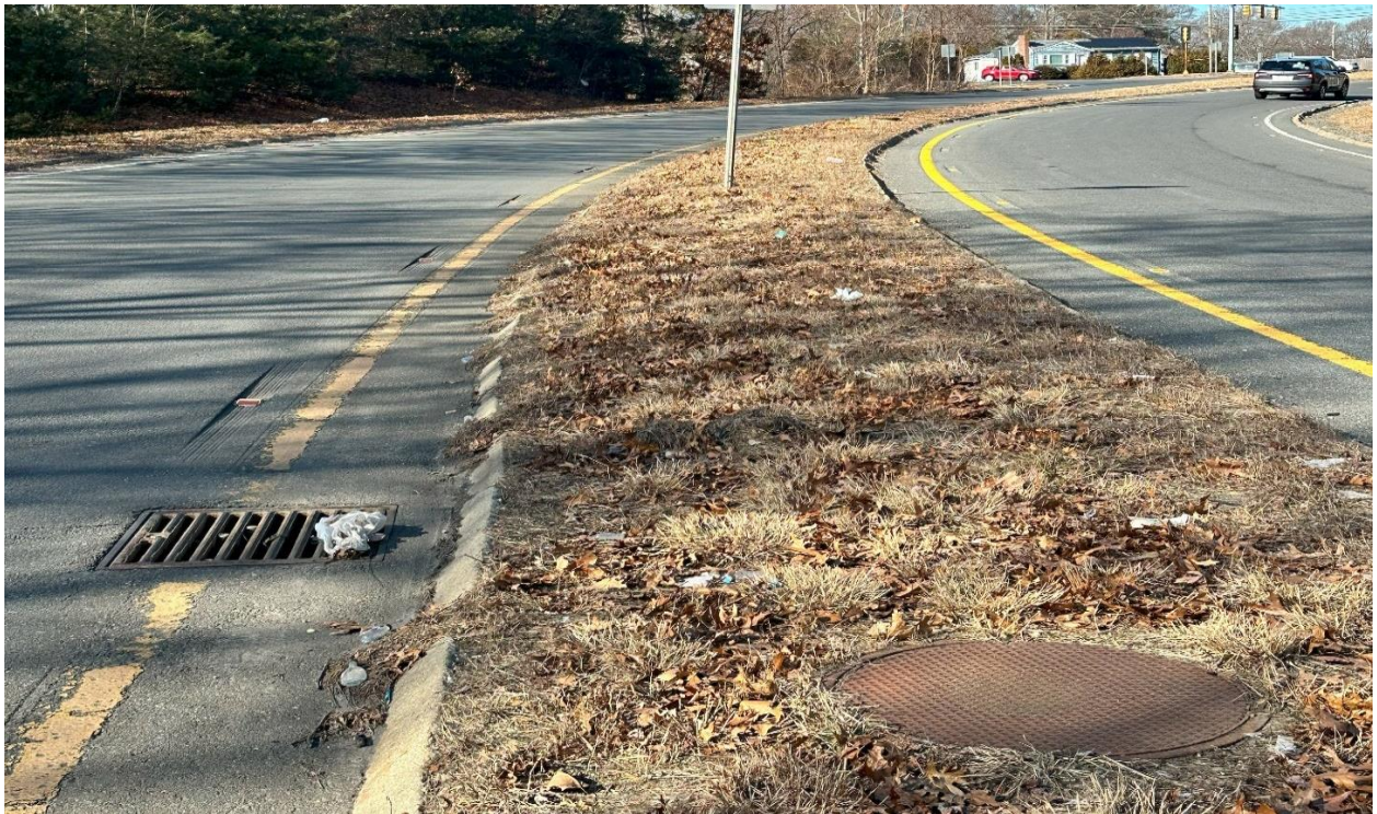
Sta. 16+00. Stormwater system 4. View looking north along Interstate 495 southbound off/on-ramp. Two catch basins located along curblines capture stormwater runoff. Stormwater flows along the ramp.
