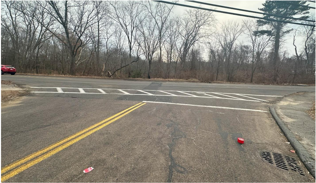
Sta. 6+40. Stormwater system 1. Four catch basins that capture stormwater located at intersection of Hartford Avenue (Route 126) and Farm Road. System 1 outfalls east of picture at the bottom of slope.
