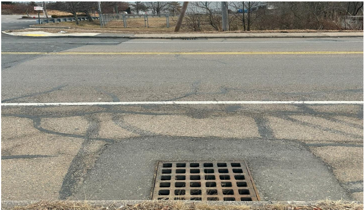
Sta. 95+40. Stormwater system 2. Two catch basins capture Stormwater runoff that flows south along the curbside on North Main Street (Route 126).
