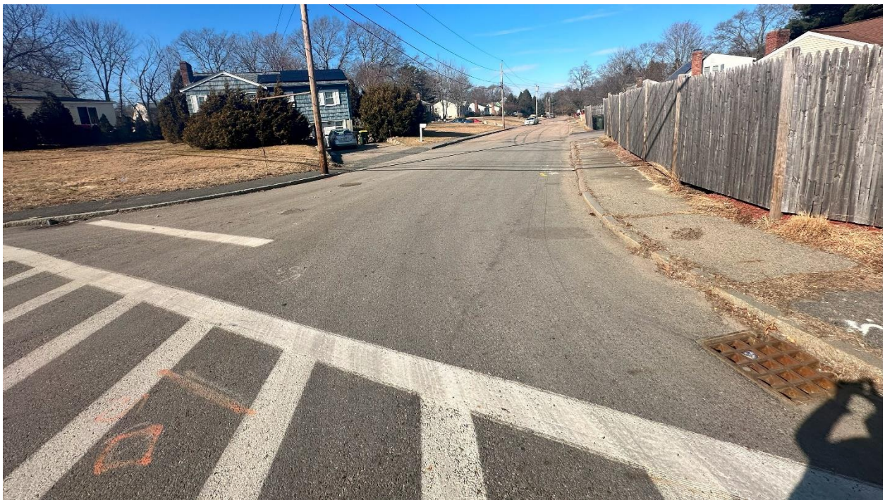
Sta. 24+00. Stormwater system 6. Two catch basins located both curb side at intersection of Hartford Avenue (Route 126) and Deerfield Lane. System 6 flows north along Deerfield Lane.
