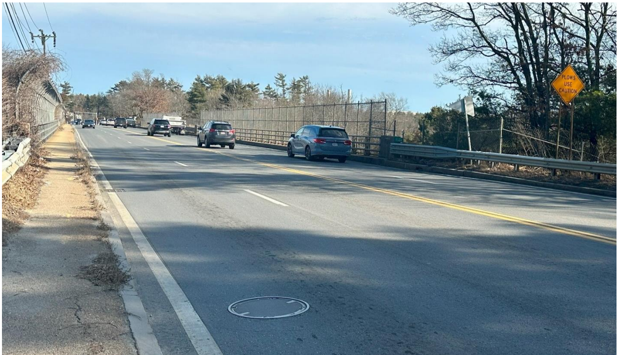
Sta. 27+00. Stormwater system 3. View looking east along Hartford Avenue (Route 126) at the end of the project. Two drainage catch basins located along both sides of the road near the bridge capture stormwater runoff. Stormwater flows north along I-495.
