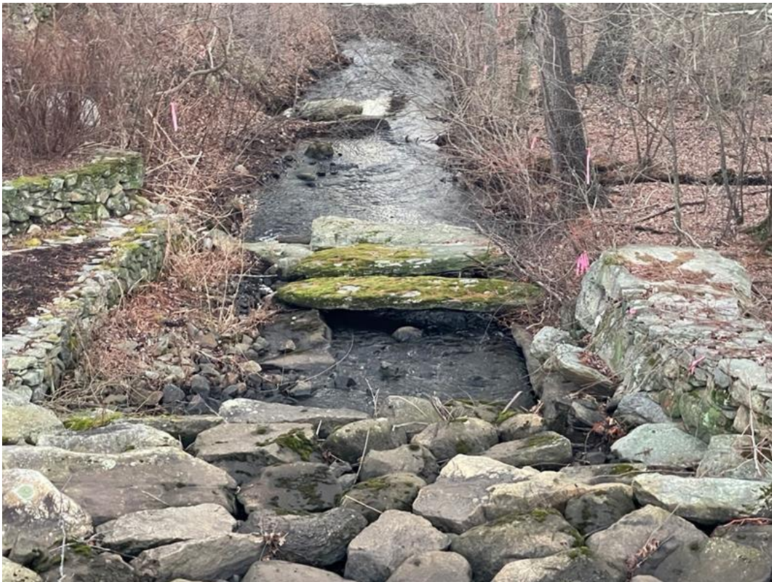
Photo No. 6: View of the stone slabs that are to be removed and replaced for the installation of the toe drain.
