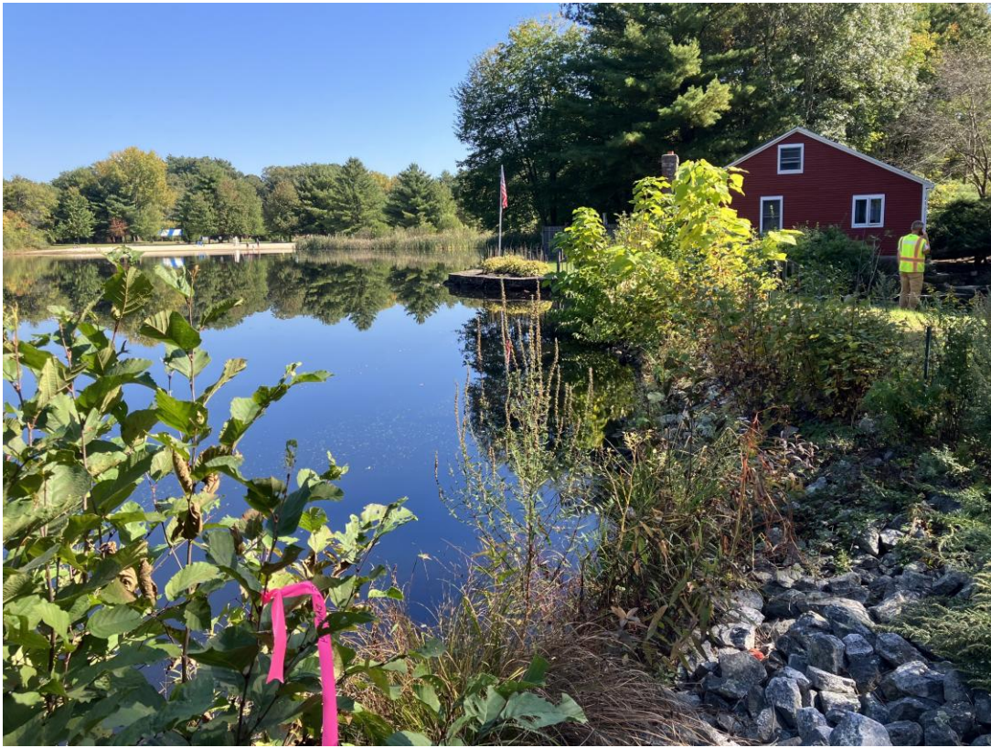
Photo No. 3: View of the southern bank of Silver Lake facing east towards the spillway at flag P-4. Notice the substantial woody growth throughout the rip rap slope.
